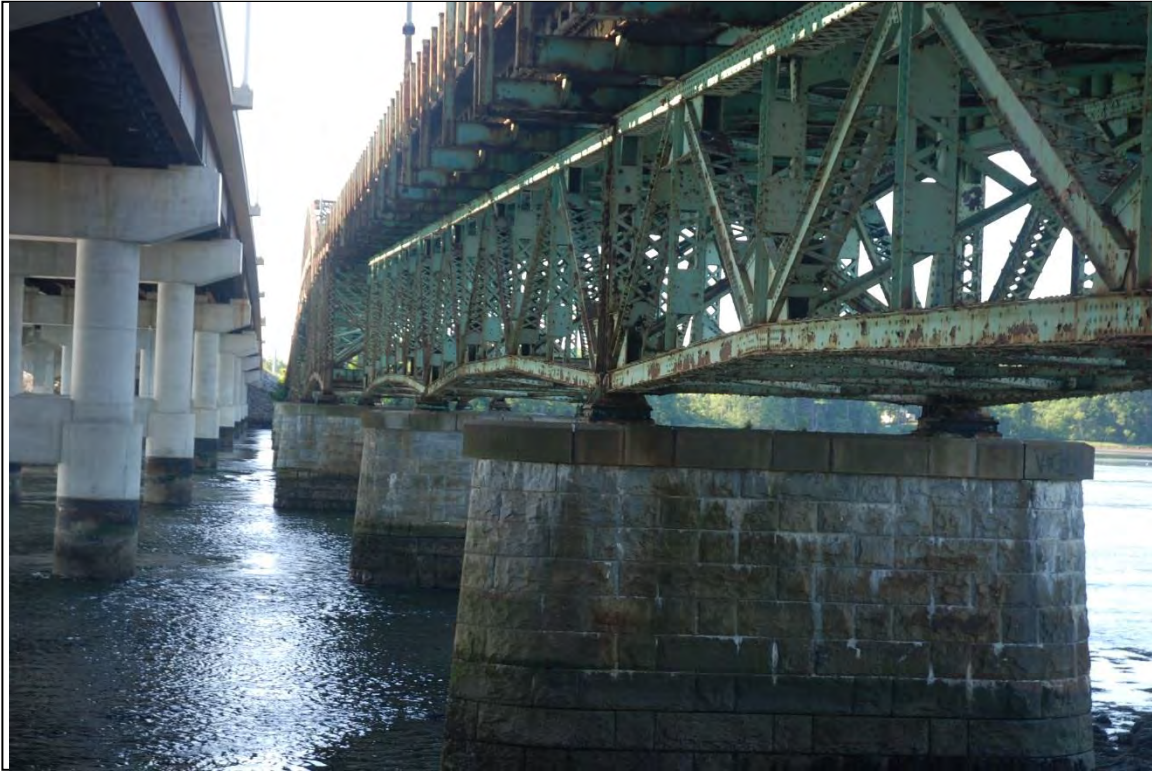
Photo # 8 Description: GSB piers (right) and LBB piers (left) Reference (file name or frame#): DOV0158_8
