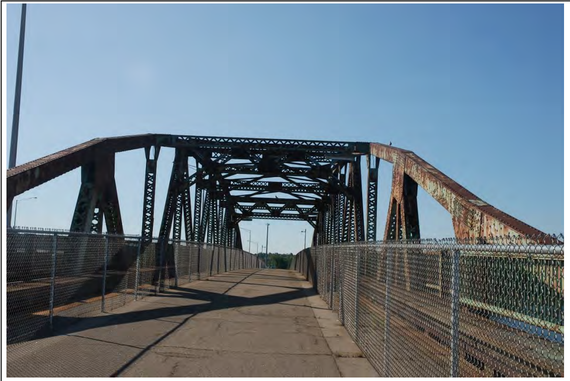
Photo # 14 Description: Closeup of center arch truss from roadway level
