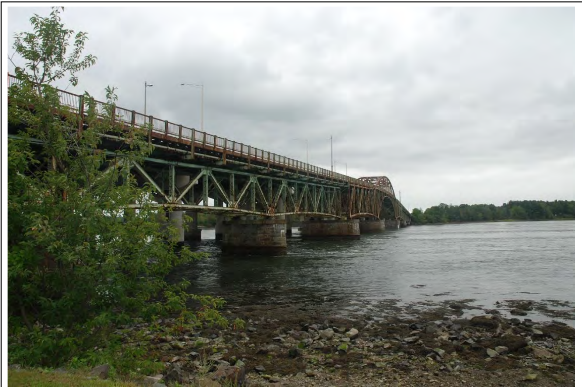
Photo # 9 Description: Overview of GSB from Hilton Park Reference (file name or frame#): DOV0158_9
