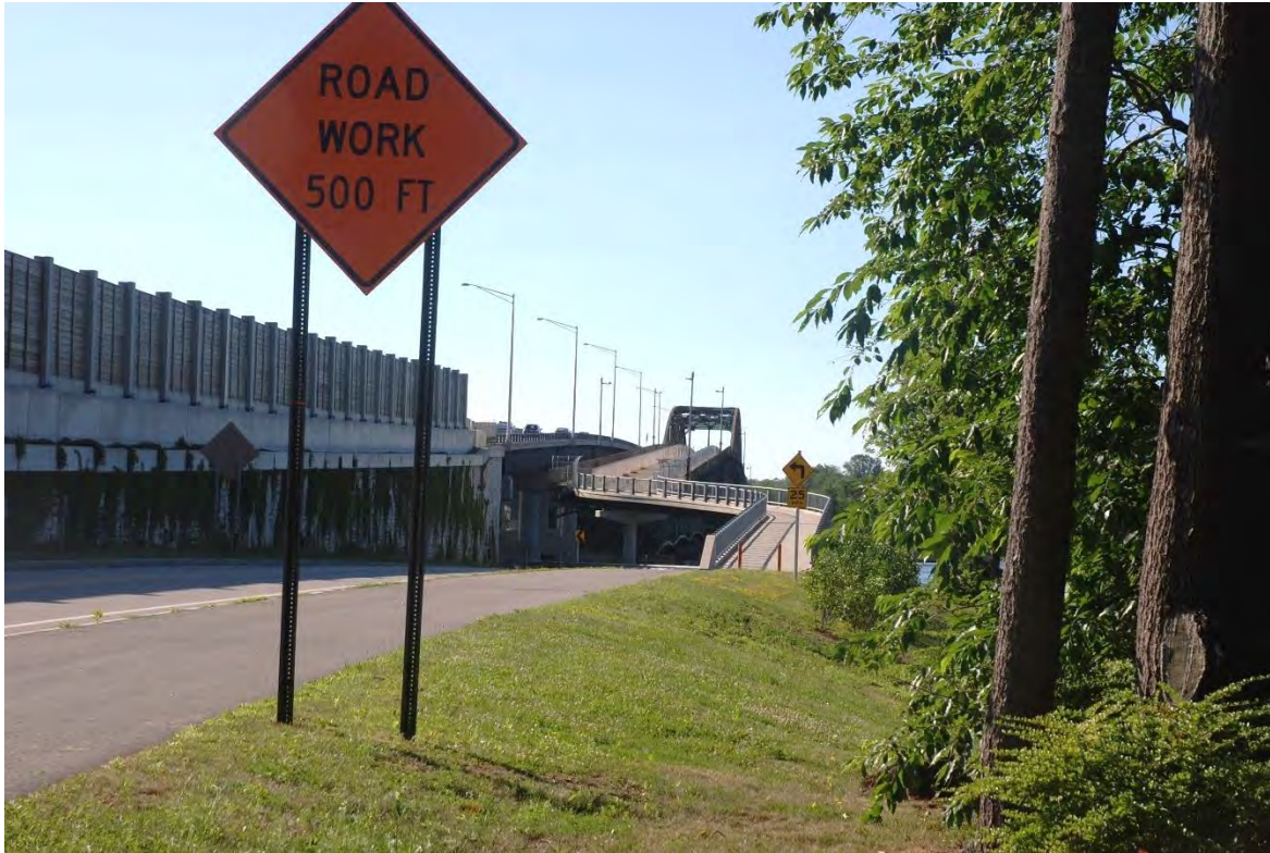
Photo # 2 Description: Overview of GSB north approach, replaced 2011 Reference (file name or frame#): DOV0158_2
