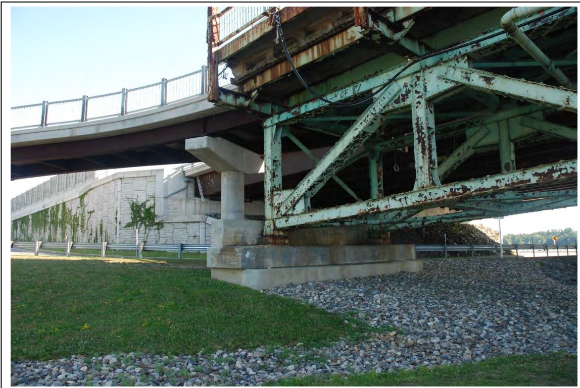
Photo # 7 Description: Detail of connection between 2011 pedestrian approach and GSB span, north abutment (water side) in center
