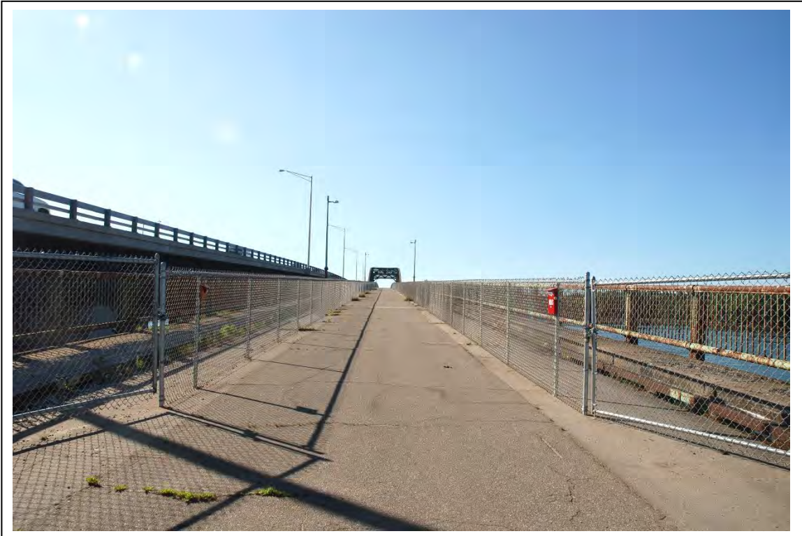
Photo # 12 Description: Overview of GSB at paved path level, showing safety fencing Reference (file name or frame#): DOV0158_12 Direction: SE
