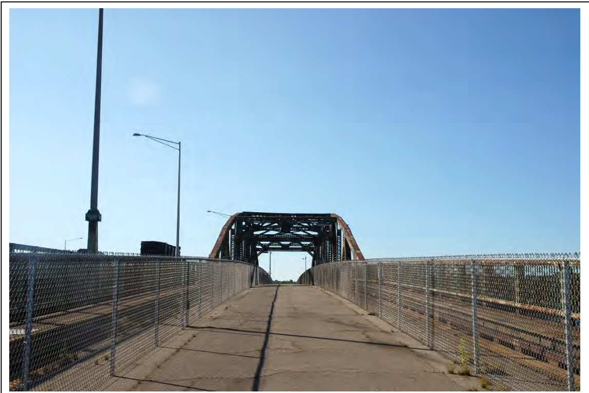
Photo # 13 Description: Center arch truss from paved path level Reference (file name or frame#): DOV0158_13 Direction: SE
