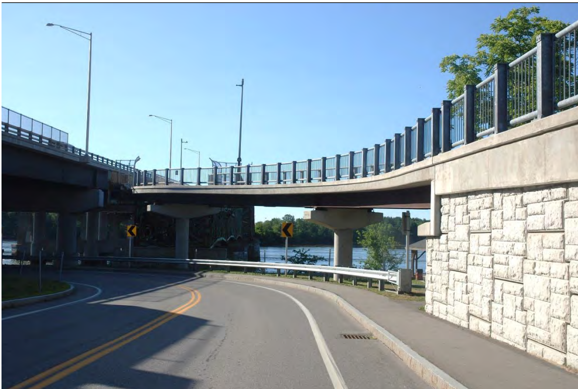
Photo # 3 Description: GSB north approach, elevated ramp on right, I-girder section in center Reference (file name or frame#): DOV0158_3
