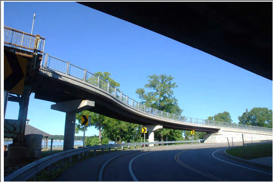
Photo # 4 Description: GSB north approach, I-girder section as seen from Hilton Drive Reference (file name or frame#): DOV0158_4 Direction: W
