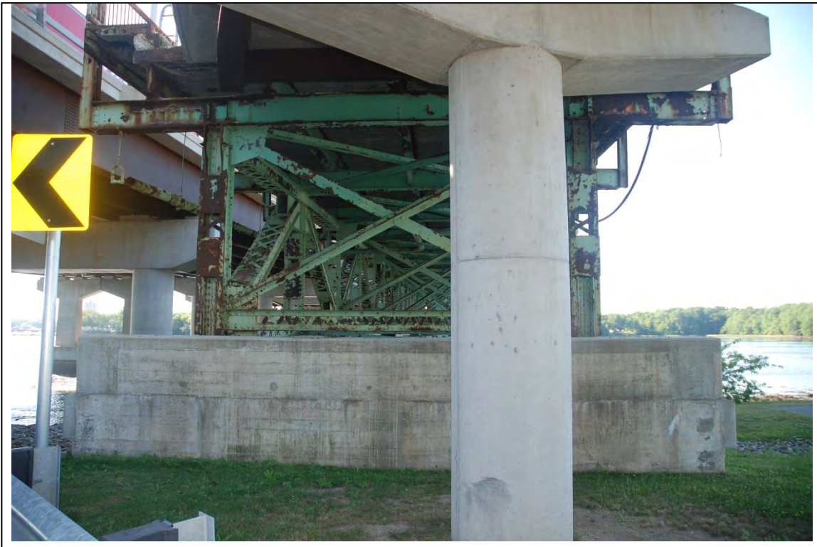
Photo # 6 Description: Back (land side) of north abutment Reference (file name or frame#): DOV0158_6
