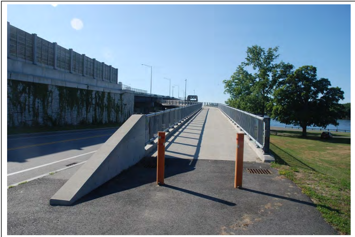
Photo # 11 Description: Entrance to north approach, constructed 2011 Reference (file name or frame#): DOV0158_11
