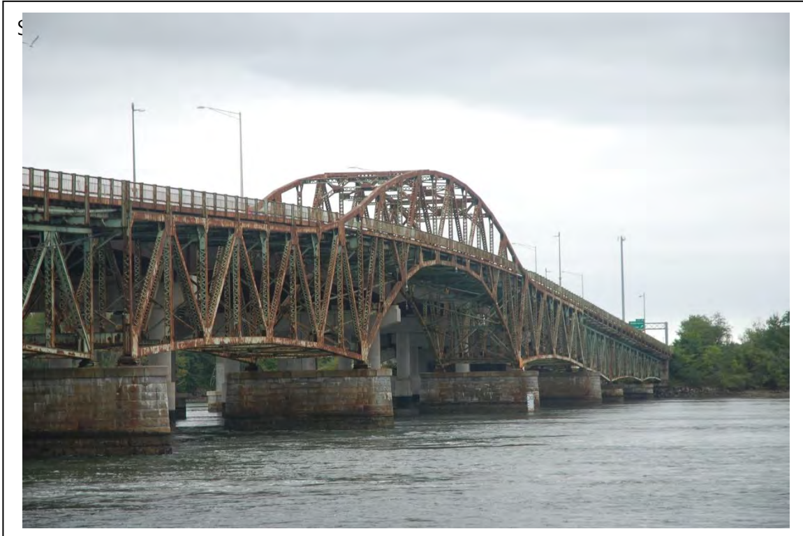
Photo # 10 Description: Center arch truss span Reference (file name or frame#): DOV0158_10
