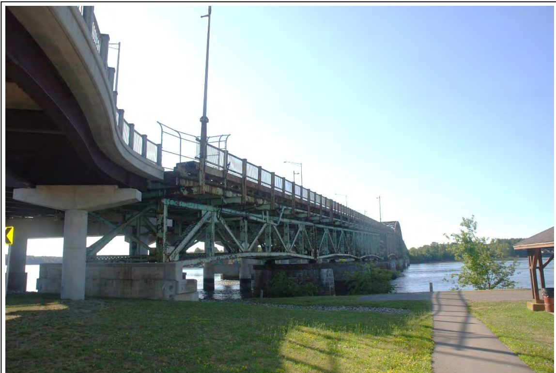
Photo # 5 Description: GSB north approach, abutment, and deck truss spans Reference (file name or frame#): DOV0158_5 Direction: SE
